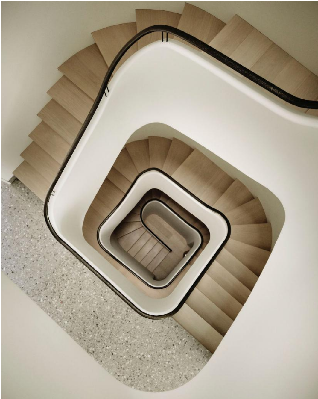
A view of the central staircase from above.
